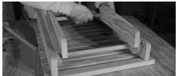
**04** Attach remaining slats (C) with glue and screws, making sure the slats are square to the stretchers and the edges line up. Use  $\frac{1}{4}$ " spacer blocks to keep gaps consistent.
